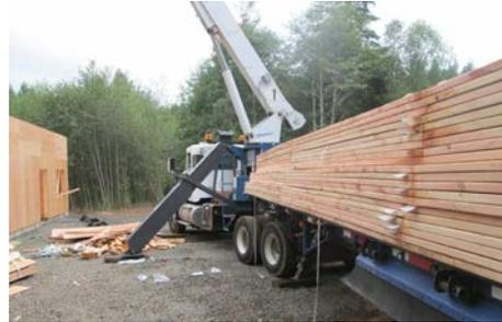
**Figure 3.** Truck-mounted crane with trusses on the trailer
