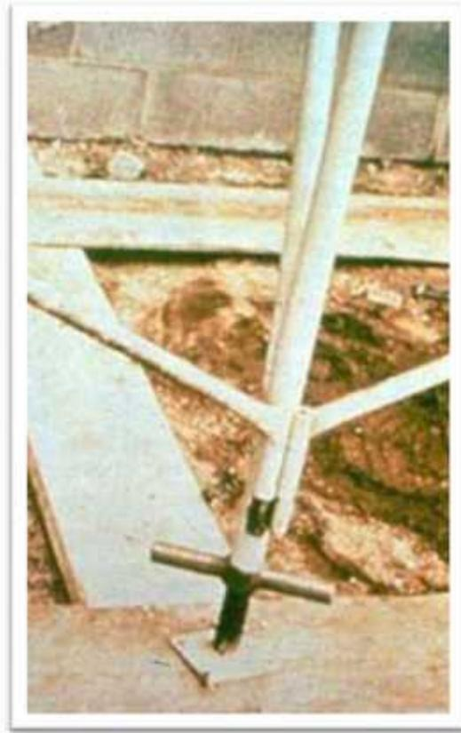
Figure 2: Proper foundation- Shows scaffold end frames equipped with adjustable screw legs and with base plates set on mud (wood) sills.
