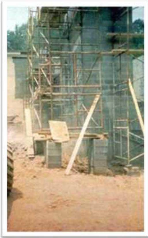
Figure 1: Poor foundation-Shows scaffold end frames, which have no base plates, erected on the top of scrap wood and unstable cement blocks.
