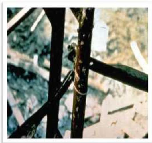
Figure 3: Poor attempt at securing cross bracing with wire.
