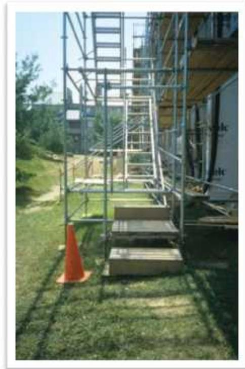
Ladders or stairways are acceptable ways to reach scaffold platforms that are more than two feet above the access point.
