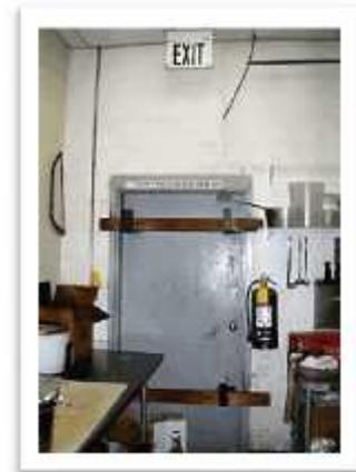
See photo at the right: What's wrong with this picture? Never hold fire doors open. The door should be self-closing, not blocked or held open!
