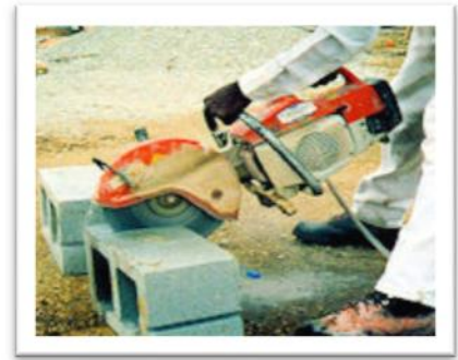
Water helps to reduce exposure to silica dust.
