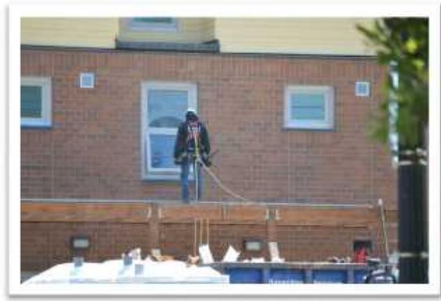
*When working at heights, make sure you are using acceptable fall protection equipment, such as the harness in this photo.*
