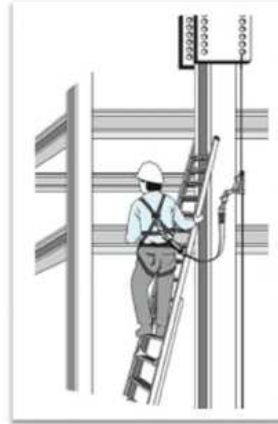
This worker is attached to a vertical lifeline with a lanyard and rope grab. The lifeline was anchored to the top of the column while it was on the ground.
