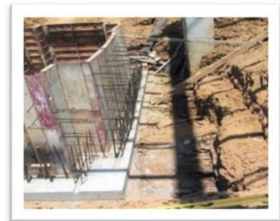
The victim helped make wooden forms for concrete pad.
