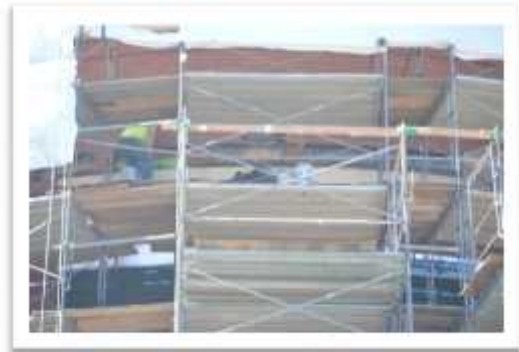
Scaffolding installation is an example of a task that should have a safe job procedure.
