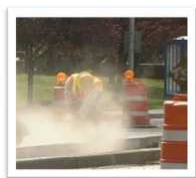
Concrete Cutting
